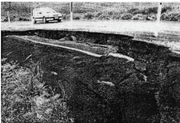
Fig. 94 (a) Slip on the Shoulder on the Road
