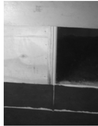
b) Driving of the sheet pile wall
