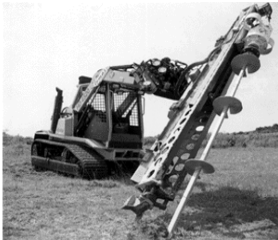
Fig. 2 Rig for the Installation of Screw Anchor
