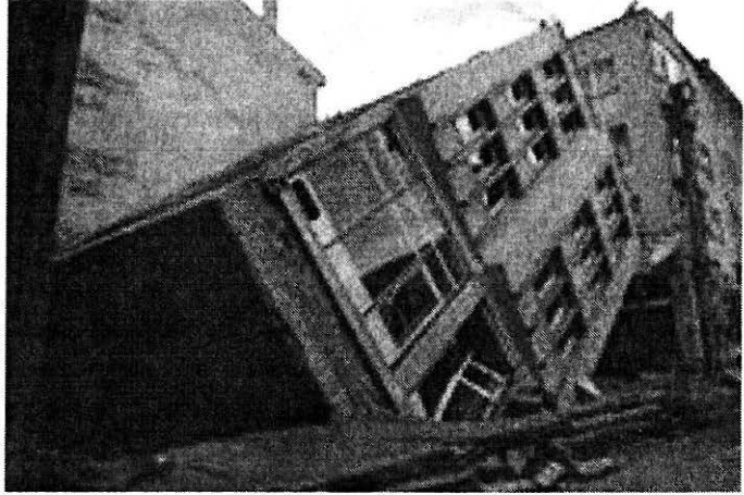
FIGURE 1 : Tilting of the Foundation with the Superstructure Remaining Intact at the Koaceli Earthquakes in 1999
