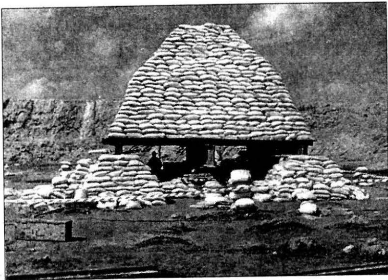
FIGURE 7 : Improper Design of Loading Arrangement
