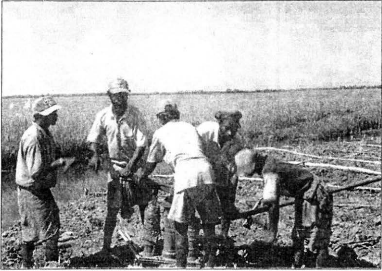
FIGURE 4 : Auger Boring with Hand Operated Mud Pump
