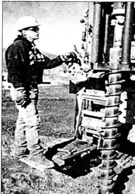
FIGURE 9 : Auger Boring with All Necessary Safety Measures
