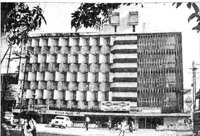
FIGURE 32 : North Face of Building Showing Tilt – Cochin
