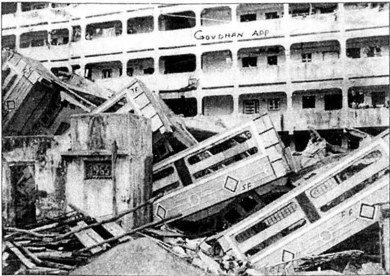
FIGURE 37 : Collapsed Building in Surat
