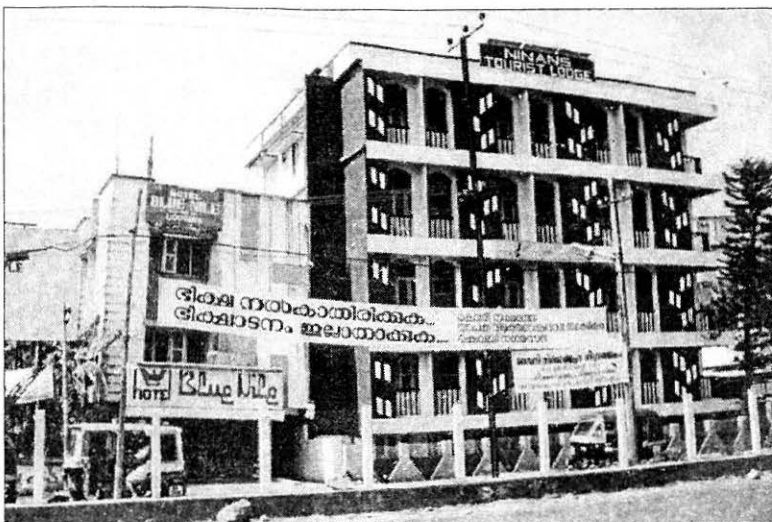
FIGURE 33 : Tilting of Other Building in Cochin
