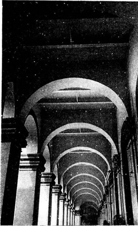
FIGURE 5 : View of Corridor with Arches
