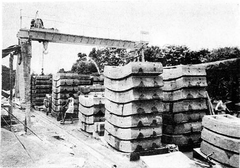
FIGURE 37 Stacks of Liner Segments ready for Placement
