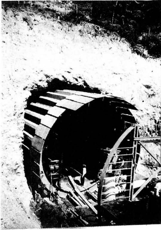
FIGURE 31 View of Blade Shield Unit at the entrance of Honavar Tunnel
