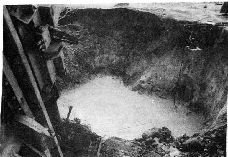
FIGURE 5b Details of Cavity at Ch. 151
