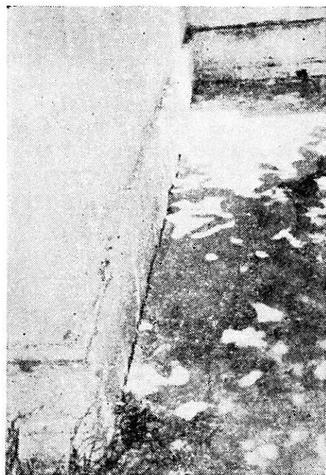
FIGURE 6 Tilting of water tank at ground level
