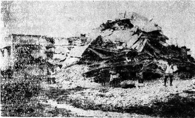
FIGURE 7 Building after Demolishing the Structure and the Neighbouring Structure on which Collapsed Building Leaned.
