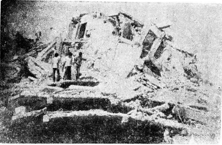
FIGURE 8 South-East Side of the Collapsed Building
