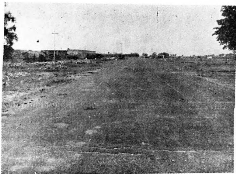
FIGURE 2 : Subgrade ready for takingover base course.
