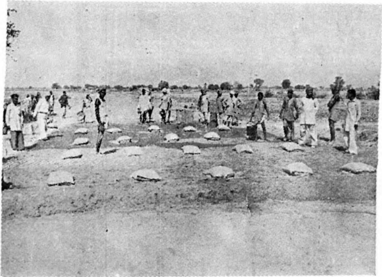
FIGURE 4 : Mixing of cement in base course soil.
